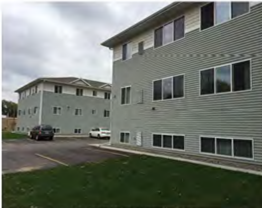
Winona West Apartments
