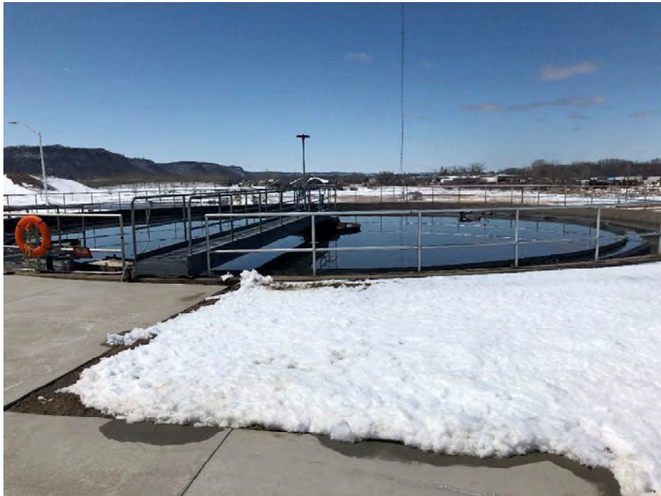
Photo 6 Primary Clarifier Tank 1
