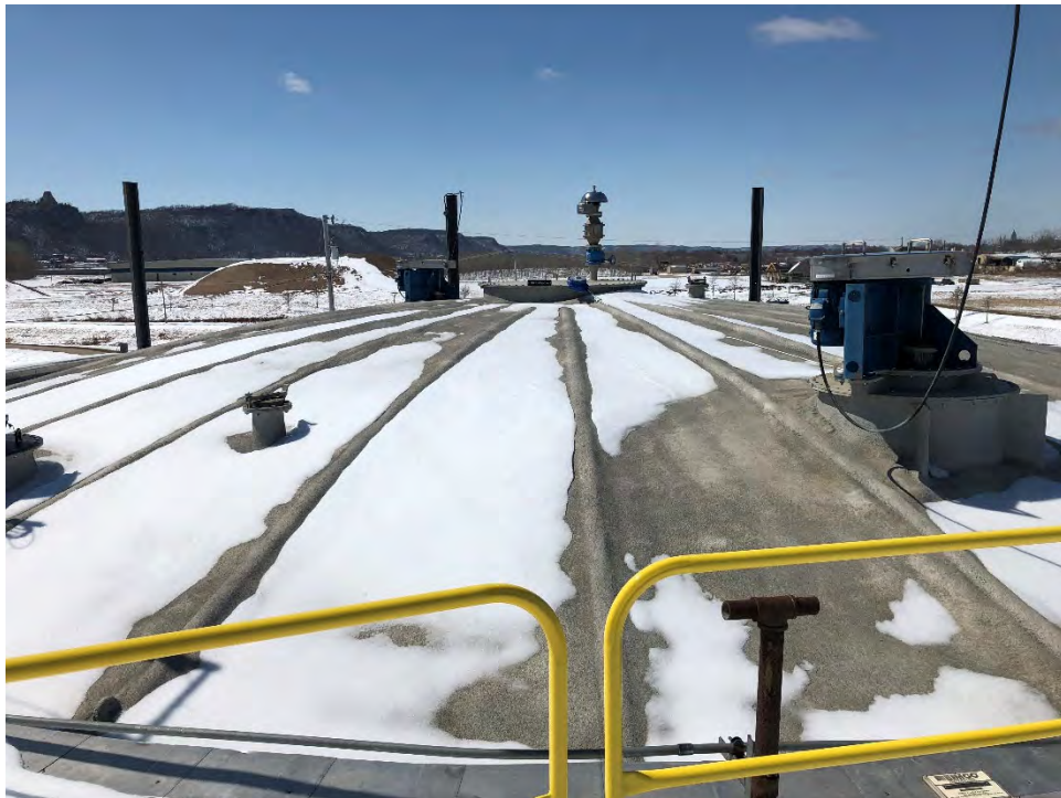
Photo 13 Primary Anaerobic Digester Cover
