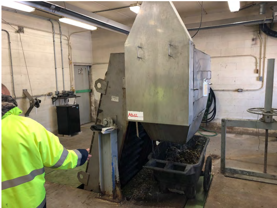
Photo 1 Preliminary Treatment Building Mechanical Bar Screen and Dewatering Unit
