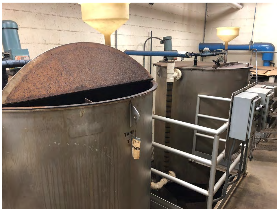
Photo 18 Polymer Mixing Tanks No.1 and No. 2
