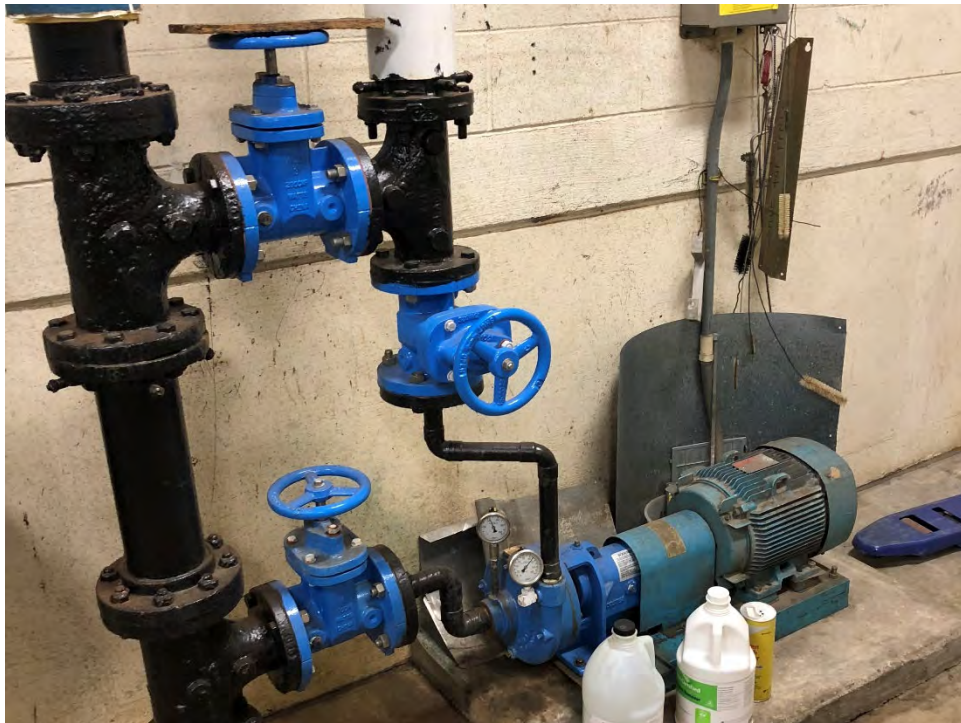
Photo 21 Wash Water Booster Pump
