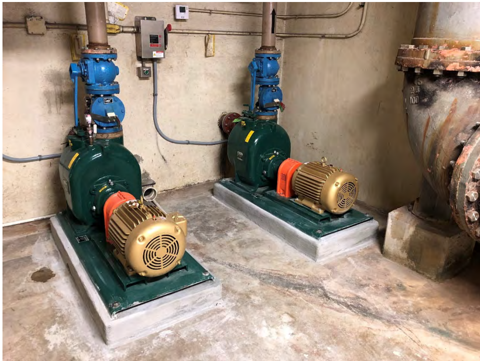
Photo 3 Preliminary Treatment Building In-Plant Lift Station Pumps
