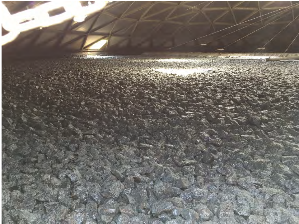
Photo 9 Trickling Filter Tank 1 Media
