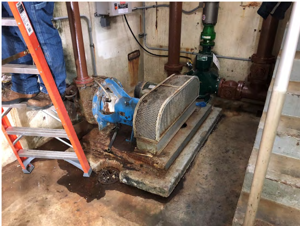
Photo 2 Preliminary Treatment Building Grit Pump
