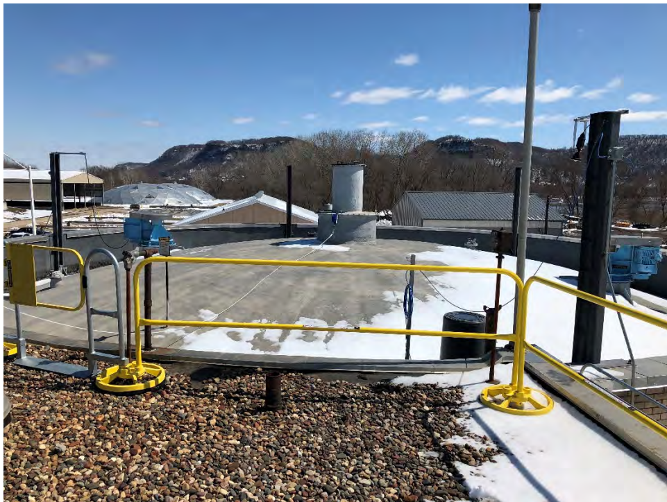
Photo 14 Secondary Anaerobic Digester Cover
