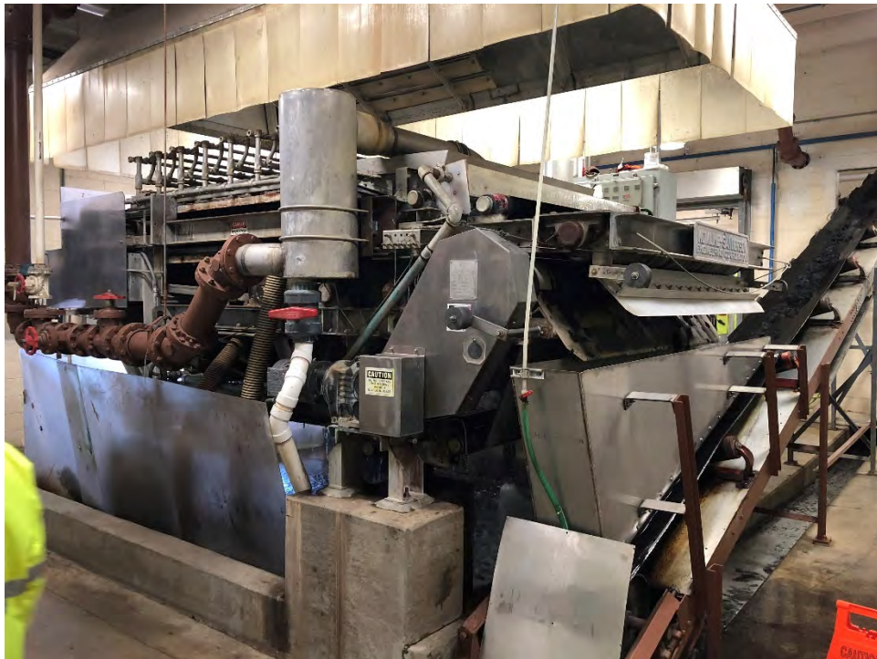
Photo 19 Belt Filter Press
