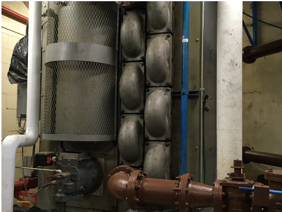
Photo 15 Combination Boiler and Heat Exchanger
