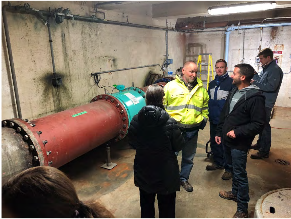
Photo 5 Preliminary Treatment Building Influent Flow Meter
