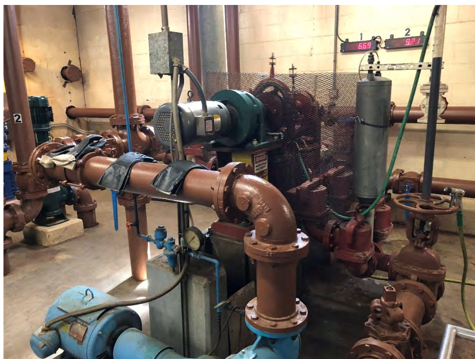
Photo 17 Digester Recirculation Pump and Grinder
