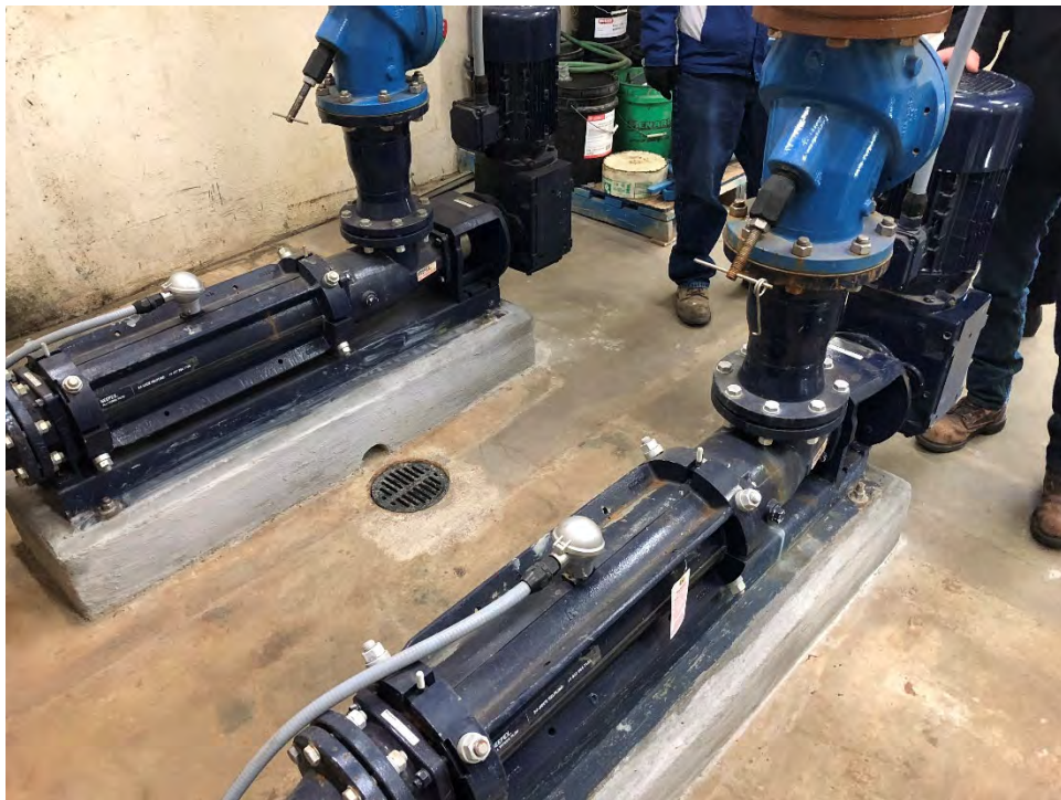
Photo 4 Preliminary Treatment Building Primary Sludge Pumps
