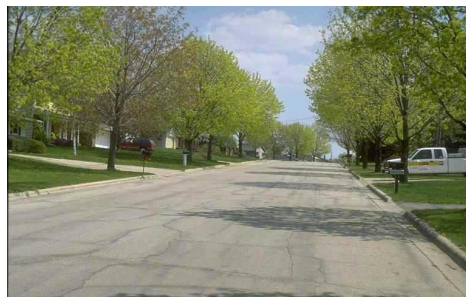
A 36-foot wide local street, especially when combined with off-street parking, creates an excessive amount of impervious pavement and tends to encourage excessive traffic speeds
