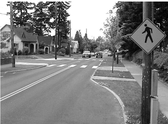
An intersection neck-down can reduce pedestrian crossing distance and slow traffic by narrowing sight lines. This design is particularly appropriate in high pedestrian areas such as near schools or parks.
