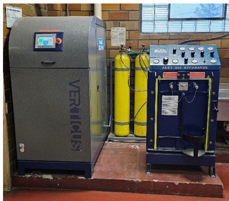
Bauer Air Compressors at Both Stations for Filling Air Bottles
